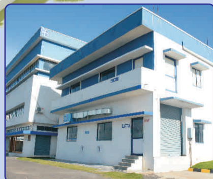
Facility Inside View
