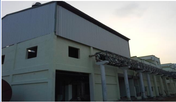
Boiler House Overview
