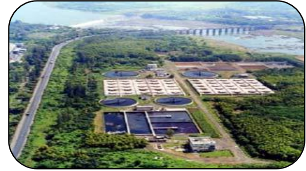
Asia's largest effluent treatment plant at Vapi with 80million L processing/day
