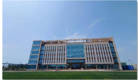
Comprehensive building (QC lab is on 3rd-5th floor)
