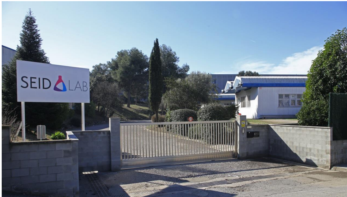
Manufacturing plant and offices
