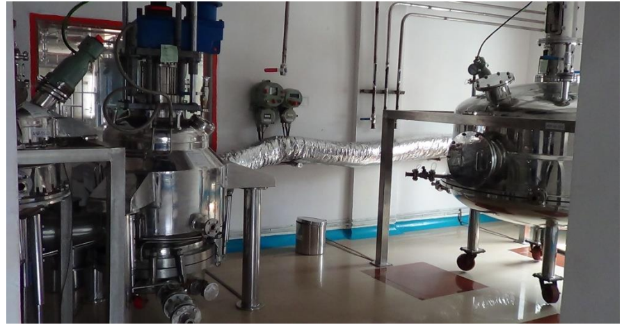
Purification Area (Ground floor)
