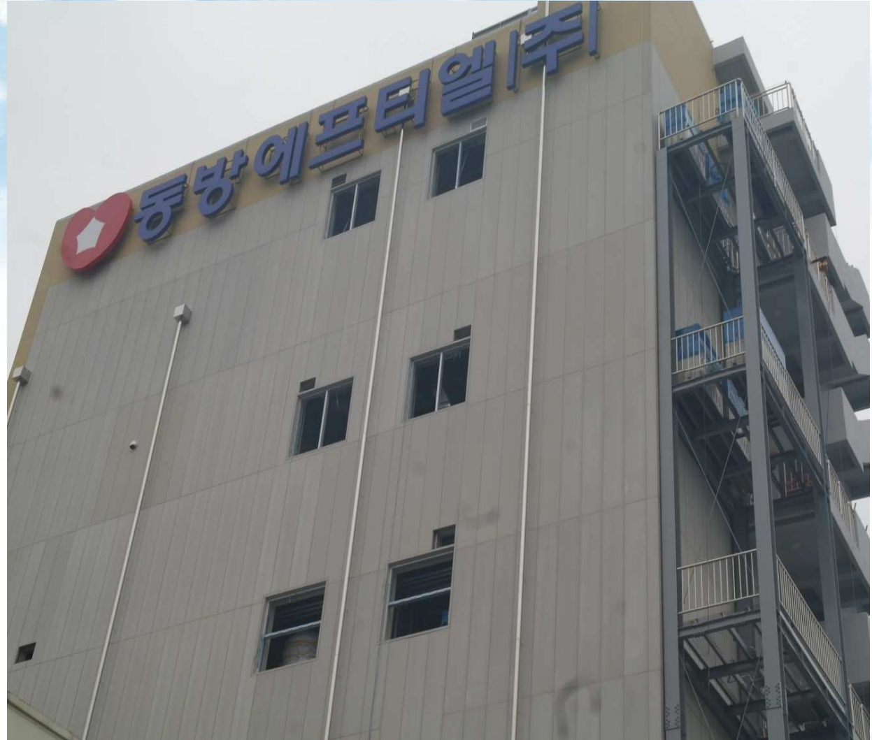
<Outside of the plant>
