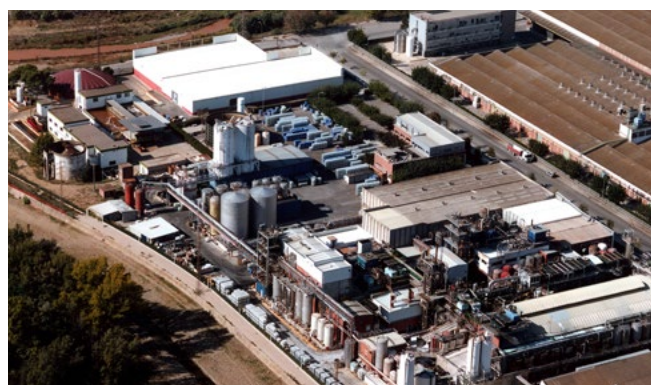
Corbion factory in Spain
